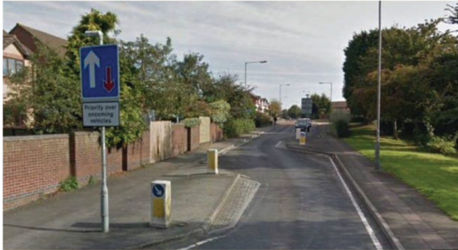
Figure 4.5 - Example of a Chicane as a Traffic Calming Measure in a Local Road
